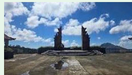
Current condition of the 3rd floor (rooftop) of Singamandawa Market
